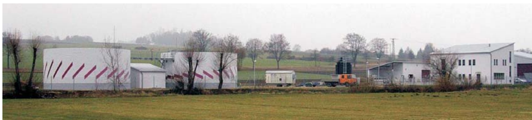
◀ View from North
